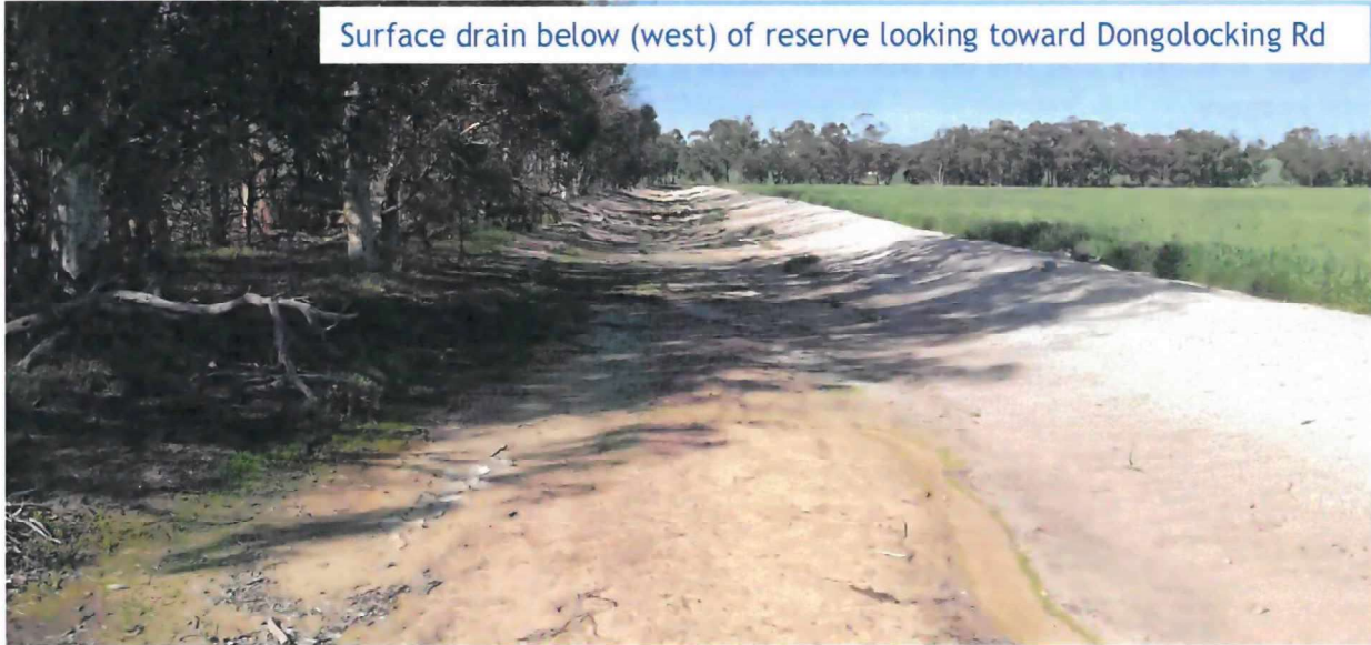
West side of reserve (no seepage into surface drain)
